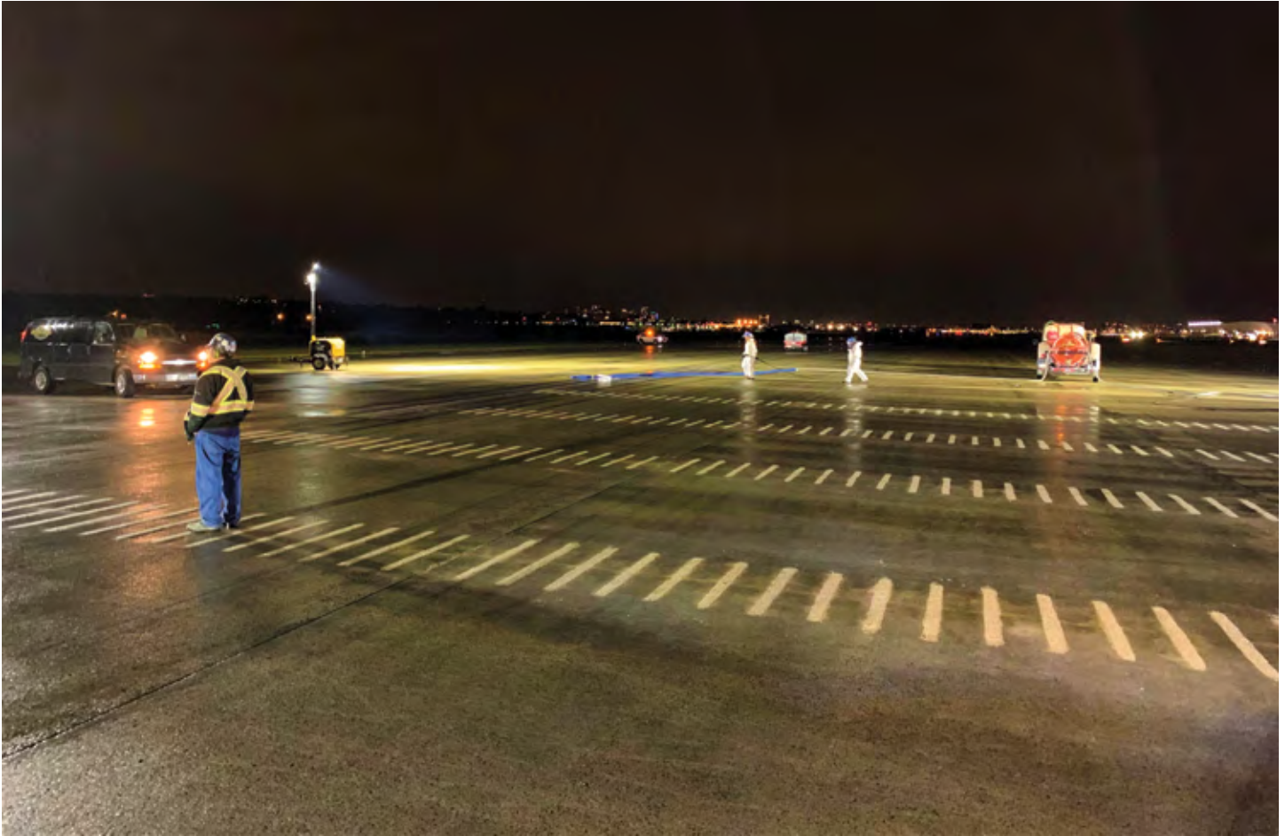
Final cleanup and inspection of runway at end of shift
