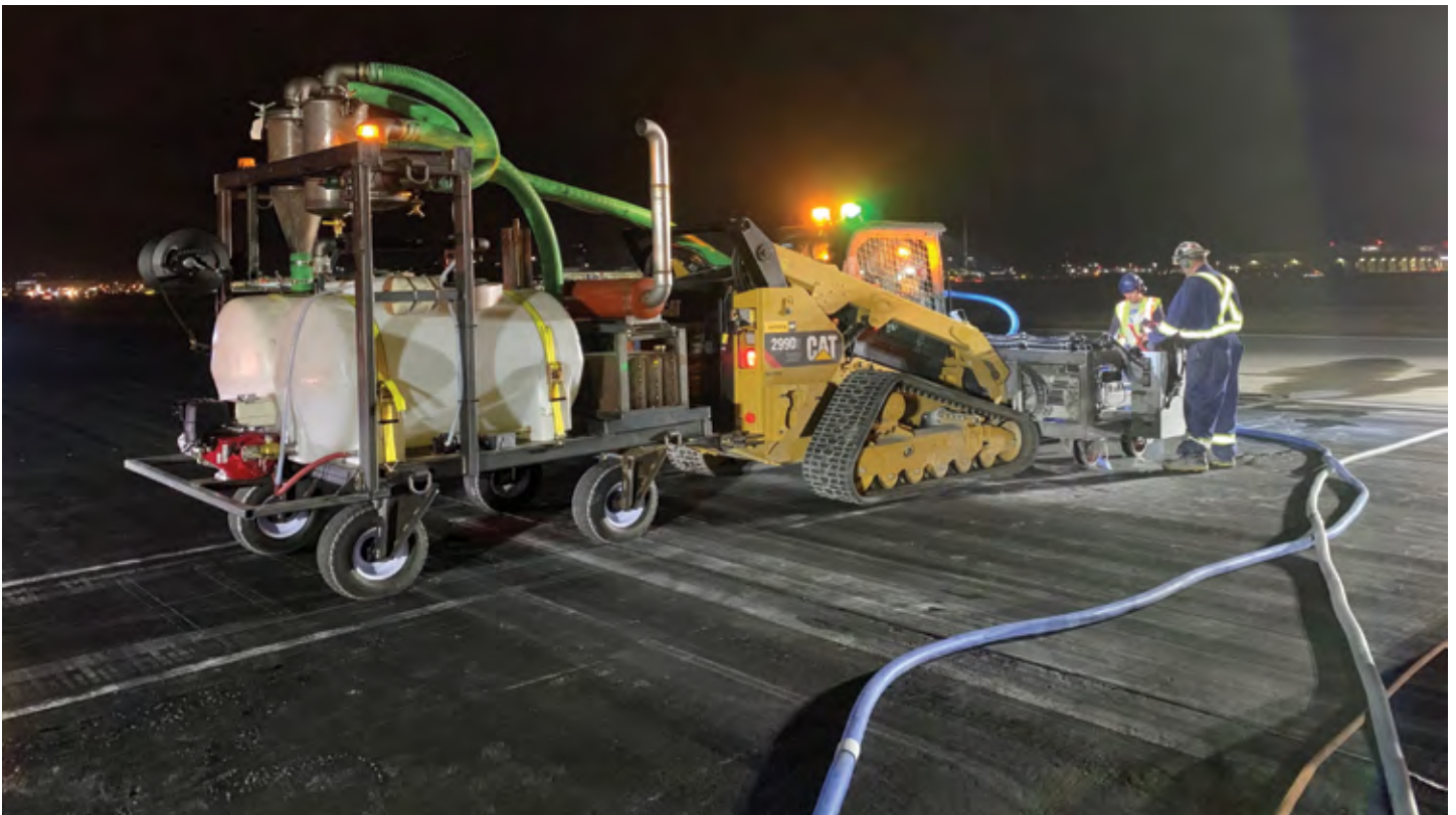
1st totally self contained, saw, skid steer and vacuum in action
