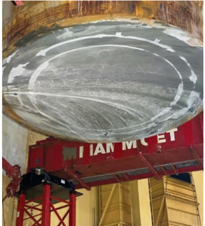
View of First Horizontal Cut - Looking at Bottom of Upper Section of Reactor Vessel
