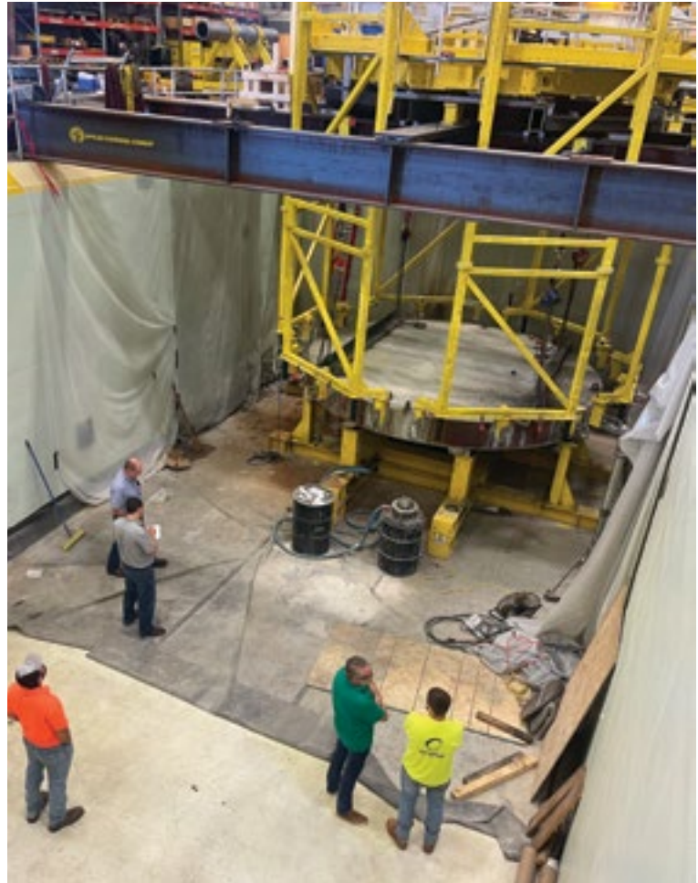
Final MPRV Platform and Pulley Supports In-Place Over Reactor Vessel Mock-Up
